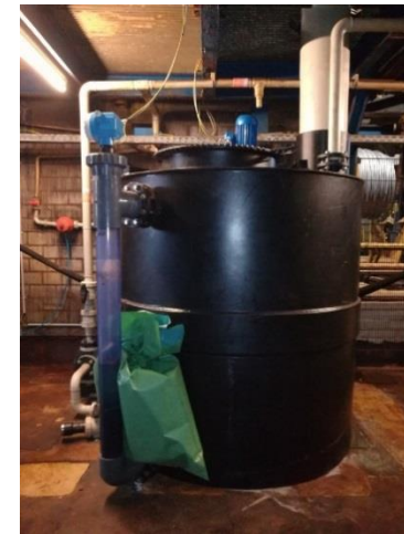
Filtration sludge storage tank
