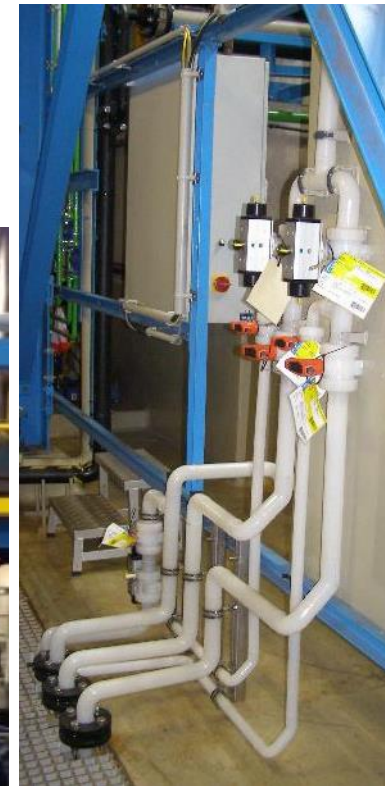
Connection to acid circulation system
