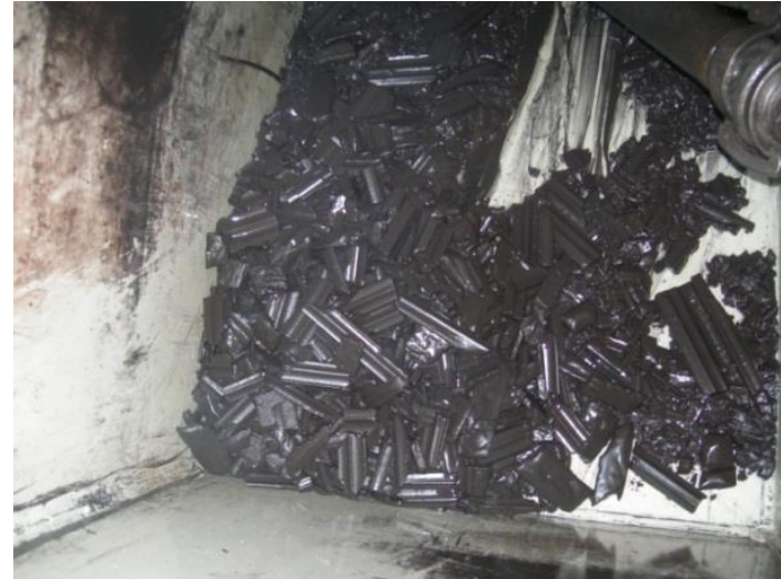
Backwash / Cleaning with solids discharged from ASRA vessel as “dry” cake, approximately 70% solids / 30% moisture.
