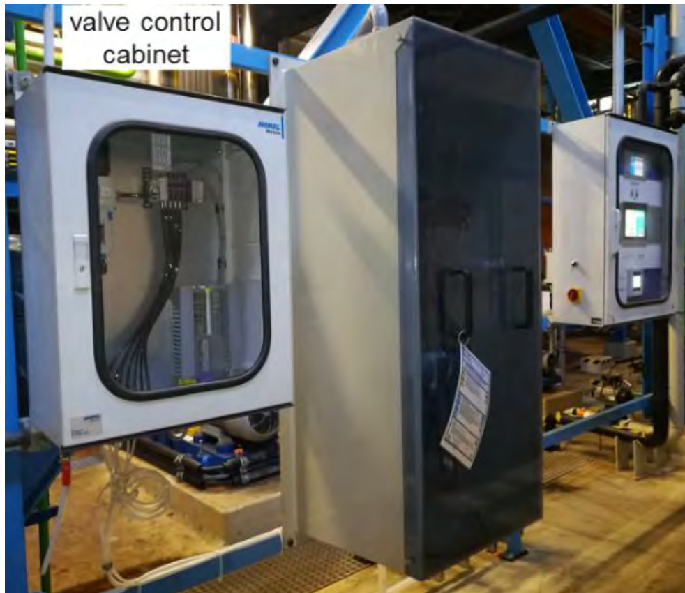
Integration of an online measuring systems at strip pickling line
