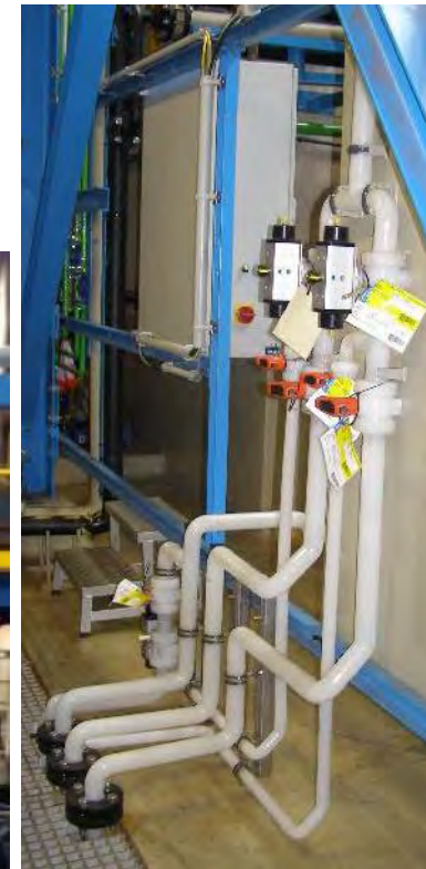
Connection to acid circulation system
